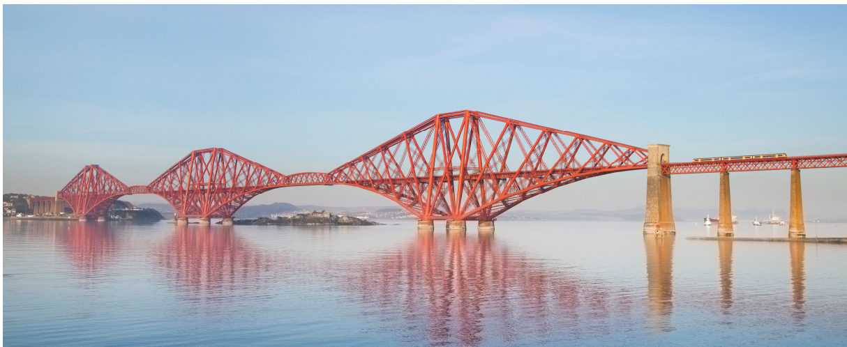
Abb. 1: The Forth Bridge, www.forth-bridges.co.uk (Foto: George Gaskin, CC BY-SA 3.0 )
